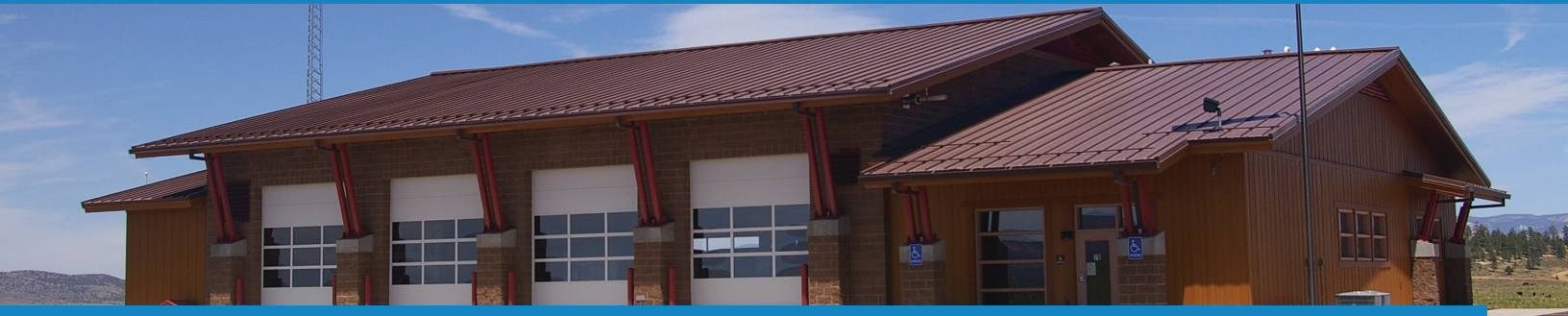
C PROJECT: UDOT Strawberry Maintenance Station LOCATION: West Valley, UT PANEL PROFILE: Double-Lok® & Artisan® Series COLOR: Champagne Metallic
