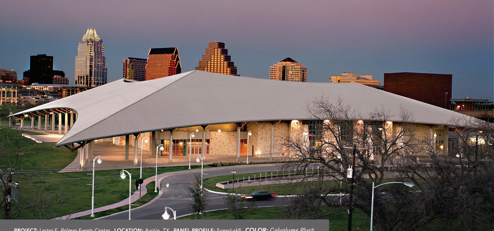
PROJECT: Lester E. Palmer Events Center LOCATION: Austin, TX PANEL PROFILE: SuperLok® COLOR: Galvalume Plus®
