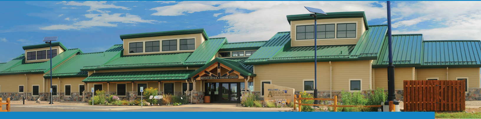
PROJECT: Audubon National Wildlife Refuge LOCATION: Coal Harbor, ND PANEL PROFILE: BattenLok® HS COLOR: Classic Green
